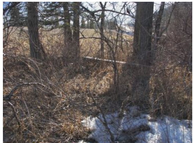
Part of concrete foundation of gatekeepers' house at site of original entrance gate to Banff National Park still visible east of Exshaw. Photo: D. McIvor
