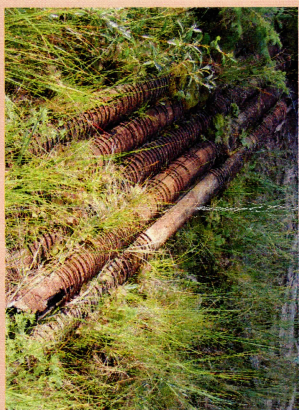
Wooden pipes that transported water from Sulphur Mountain's thermal springs to facilities downhill can still be found. "Lithia water" was once bottled for its potential curative properties derived from the Middle Springs. Photo: H. Dempsey
