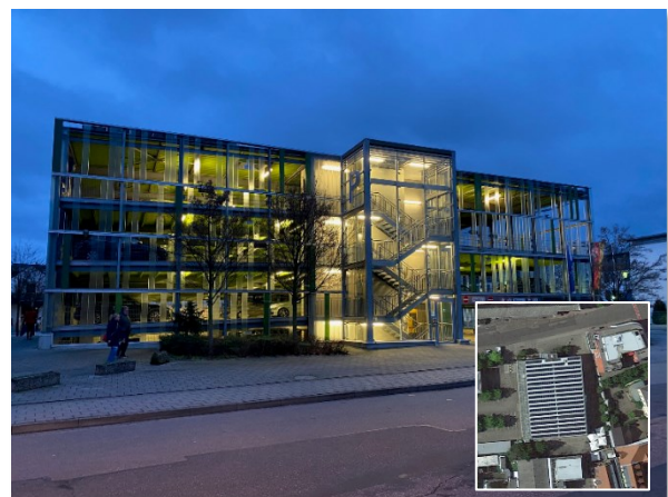
Parking structures need not be massive concrete structures, as this steel frame structure demonstrates, and have environmental management advantages over open surface lots. Inset photo shows the roof of this structure apparently covered in solar panels.
